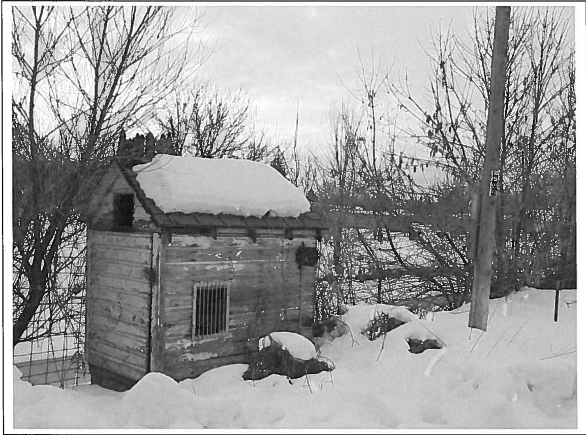
Nevada Street Pump 97-P 01/28/2004
