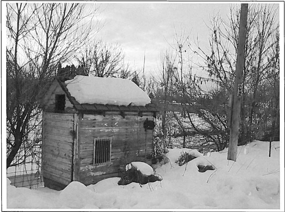
Nevada Street Pump 97-P 01/28/2004
