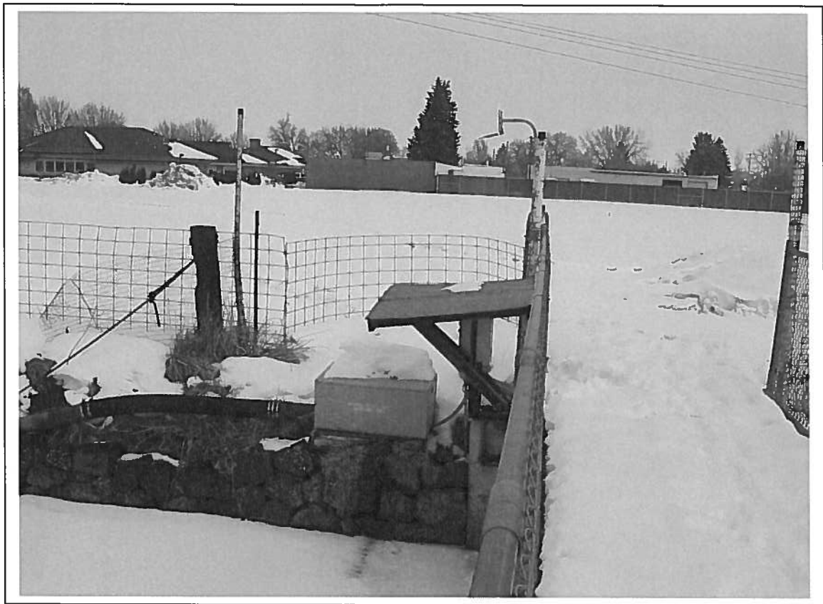
School Pump 01/28/2004 Tag No. A0011706
