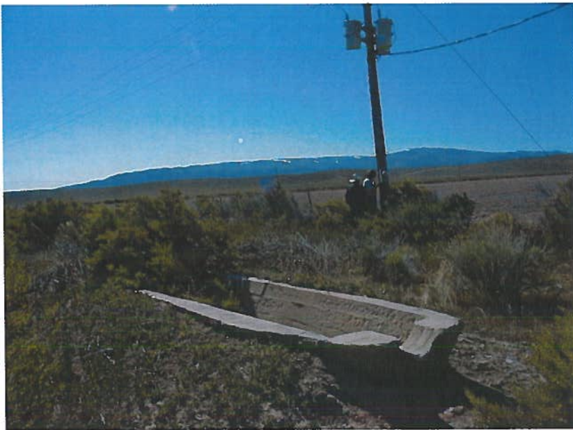
10. Old concrete ditch in T16S R24E section 23 that was originally used to convey the water by E. Bruce Durfee. Looking Southeasterly.
