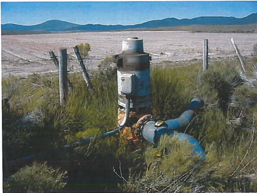
8. Bruce Durfee's pump in T16S R24E section 23. Looking south. Site tag A0004513. GPS file name A0004513.
