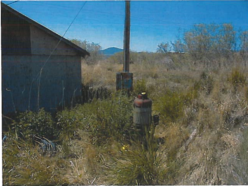
19. T16S R24E S12 North pump.
