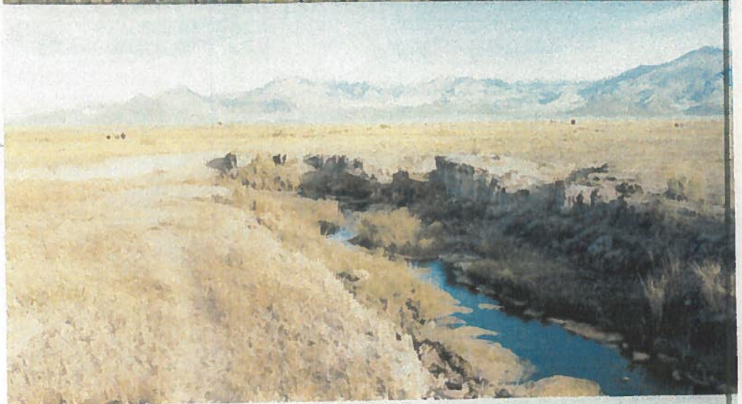
POINT #8 WEST OF EARTHEN DAM
