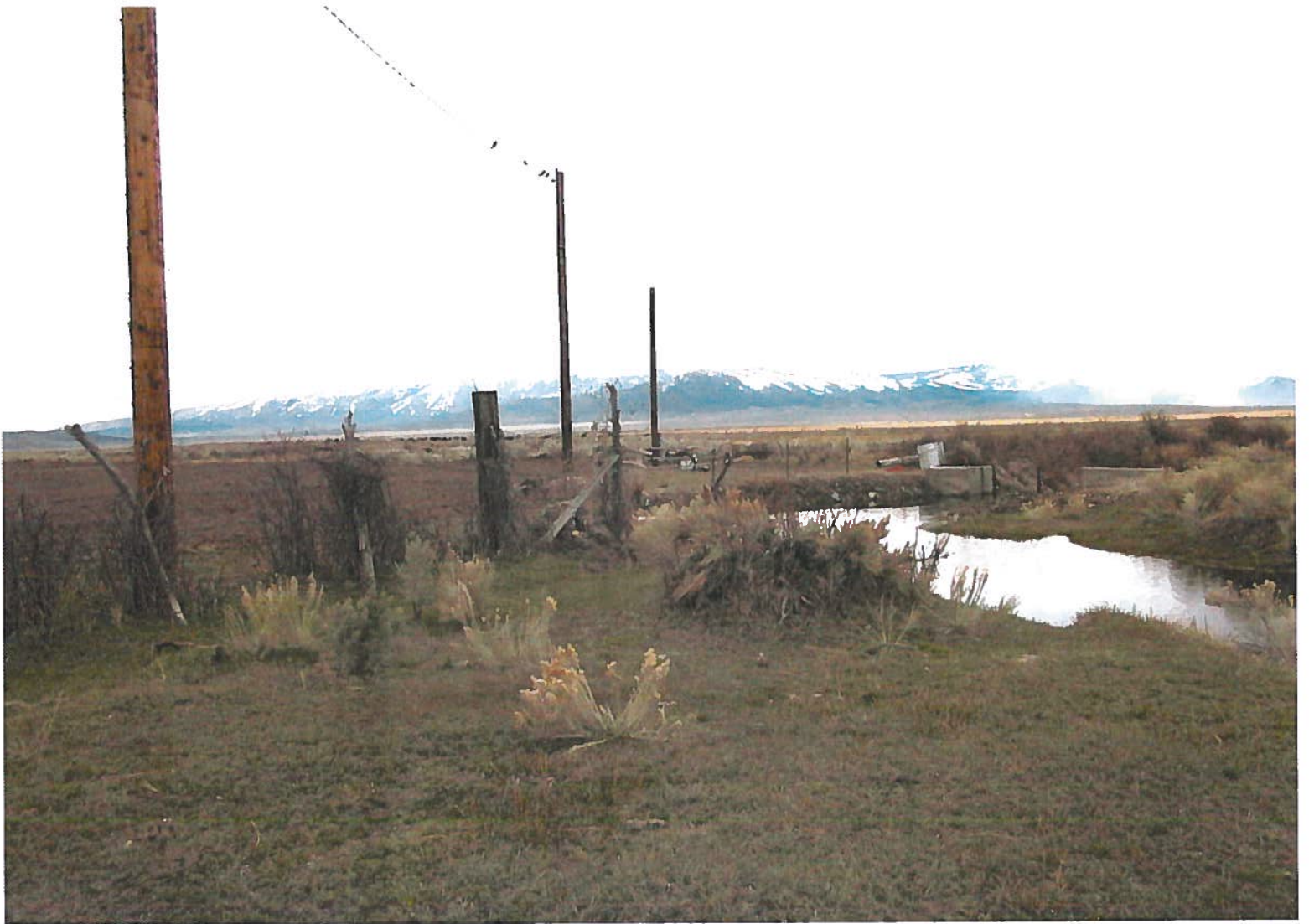
Looking from upstream at diversion & new pump.
