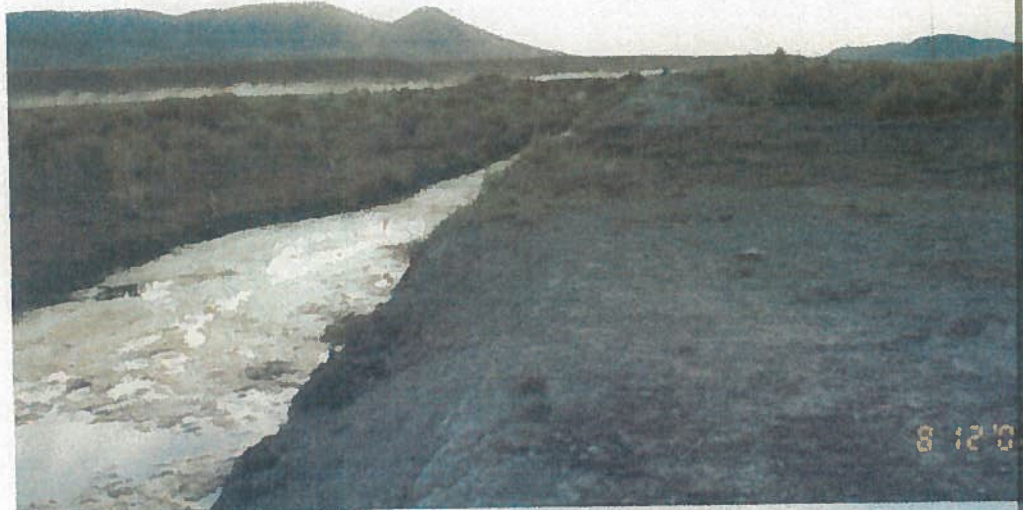
POINT #1 EARTHEN DAM LOOKING WEST EAST
