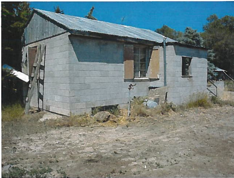
Figure 7. POD. The pump is located in the basement of this building.
