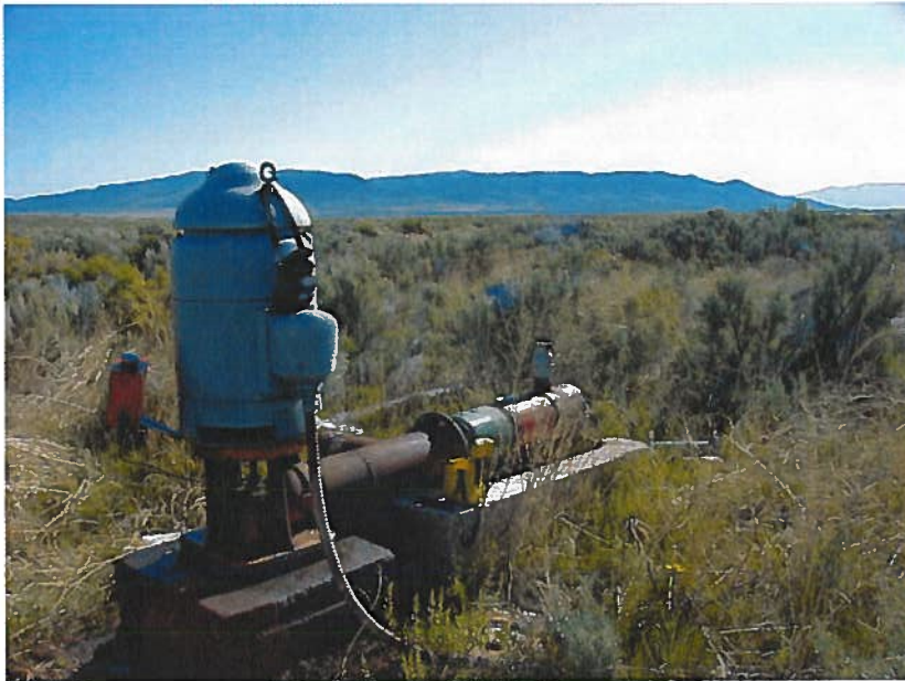
3. Looking Northeasterly at Kent Durfee's POD in section 14.
