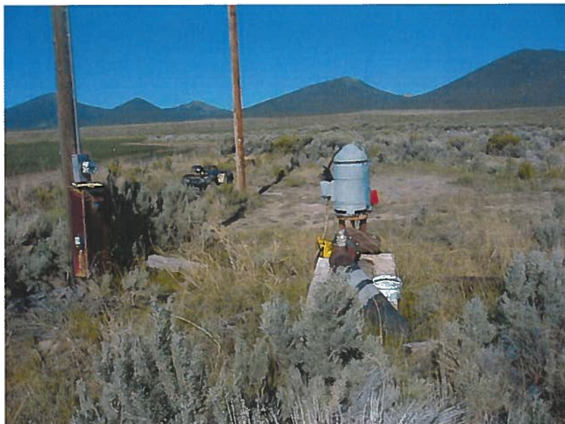
4. Looking Northwesterly at Kent Durfee's well in section 14.
