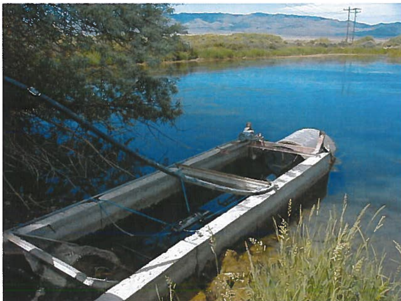
Figure 6. Close-up of the concrete structure in the C Bar (Arimo Corp) pond.
