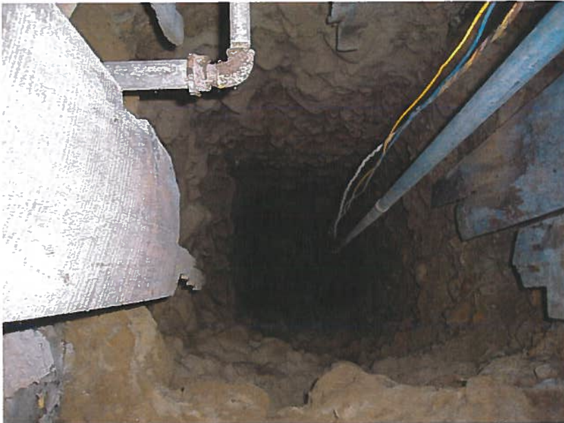
Figure 9. Looking down the hand dug well in Naf.
