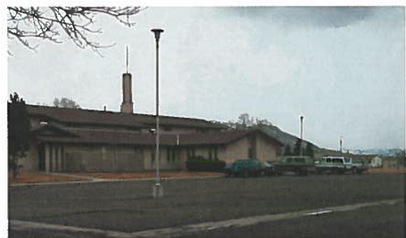
Photo 2. Looking northwesterly at the southeast corner.
