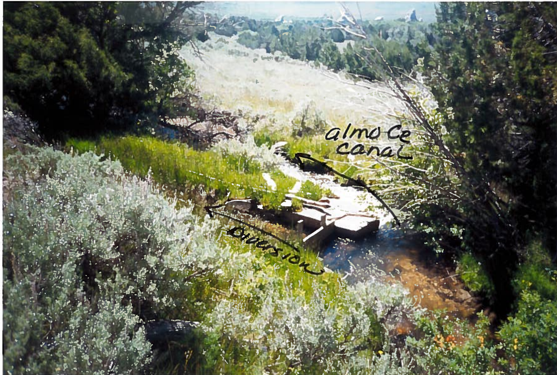
Almo Creek Diversion from Almo Cr main canal.
