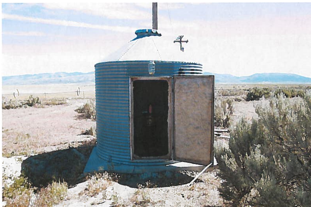
Figure 2 Looking into the well house. GPS file CROOKPOD.COR site description "Pole 28033"
