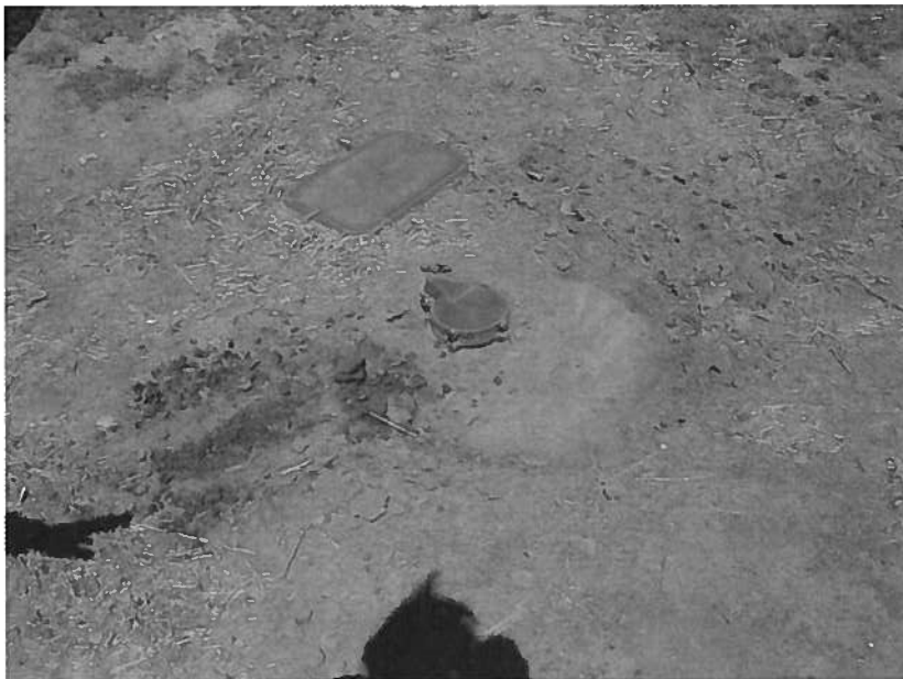
Hal Anderson A43-04024A, T14S R27E 8 SESENE. This well was previously used for irrigation. After caving in the well was converted to a domestic well. The well is located south of the Anderson home. No site tag. GPS file name t053120a.
