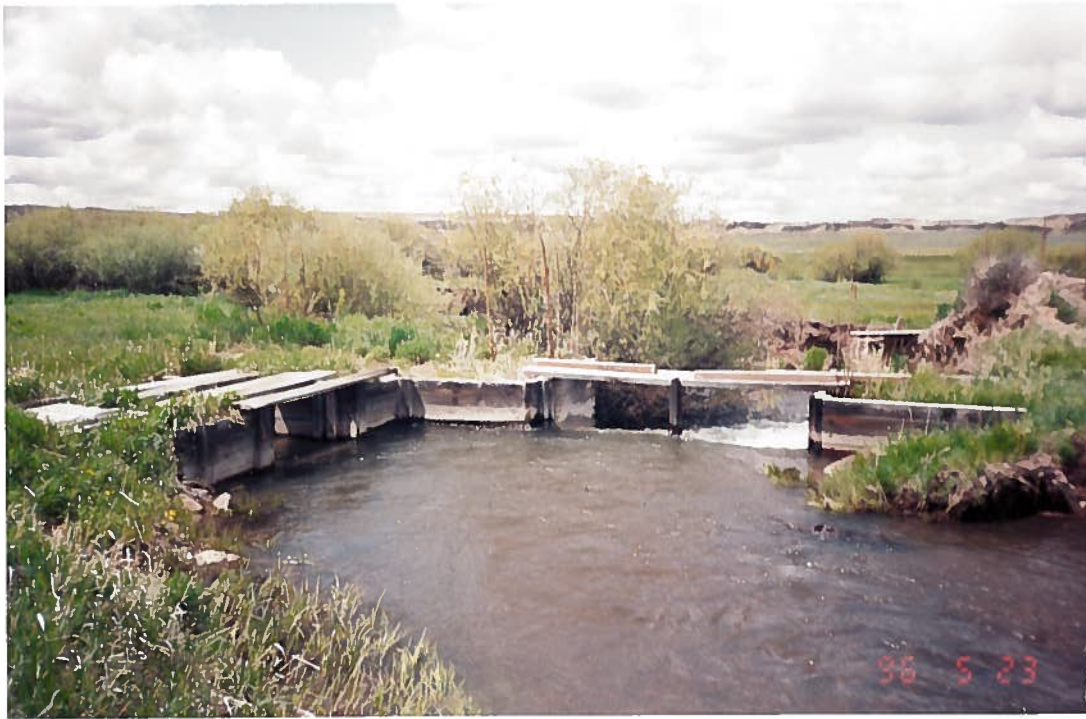
POD NO 7 Ditch on left side of photo
