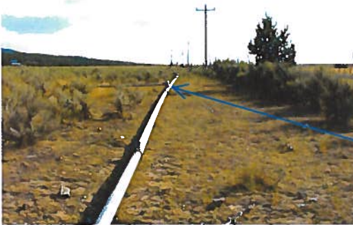
File:43-2532F mainline look s
