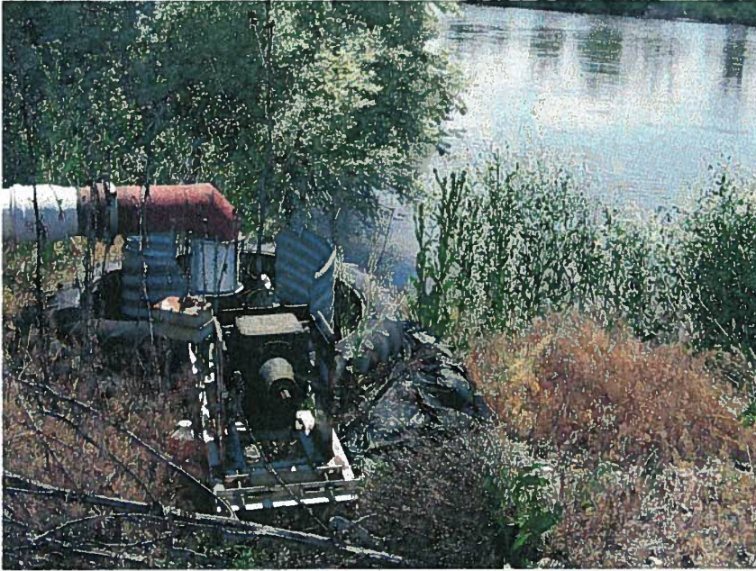
A0017651. Pump is run by tractor. Picture taken facing west. Pipe where water runs eastward to open ditch is visible in left middle of picture.
