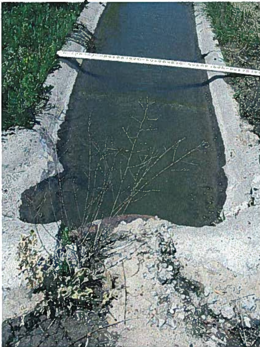
Photo taken of ditch about 10 feet downstream of where Snake River pipe would flow into ditch system. Culvert can be seen in lower middle portion of picture. Photo taken facing north. From here, ditch runs north according to attached ArcView layout. Dimensions of ditch in field exam report. Water in the ditch was Hurd Gulch water, but was used in measurement to assess capacity of ditch. According to claimants Robert and Gerald Henggeler, water from Snake River is meant to supplement Hurd Gulch water when that water runs low.
