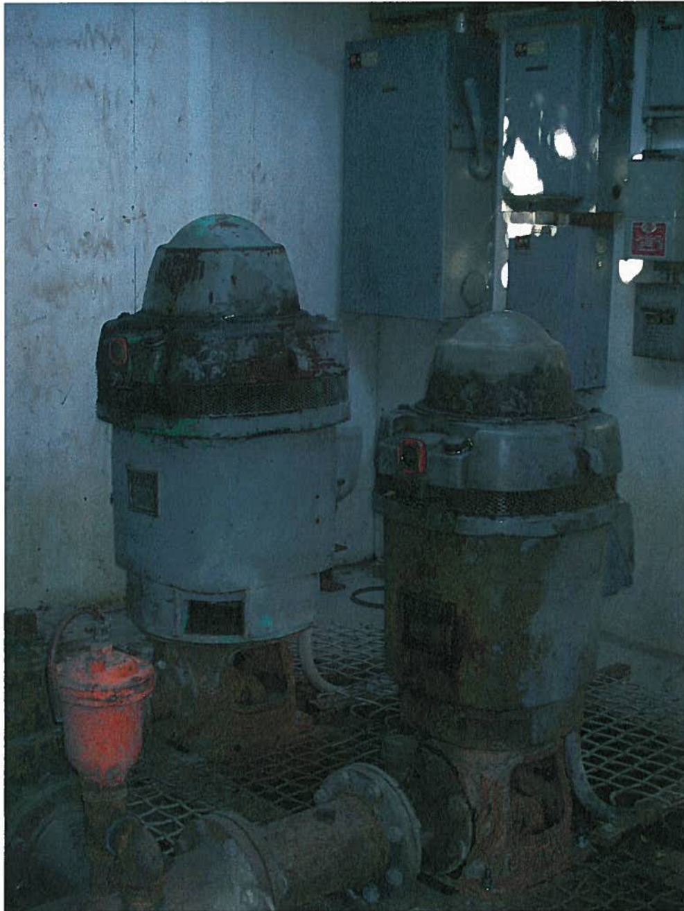
Snake River pump site for 3-2013 and 3-7007. Pump for 3-2013 is 100-hp pump on left and pump for 3-7007 is 60-hp pump on right. Picture obtained 3/4/06 on Lewiston field exam. JD
