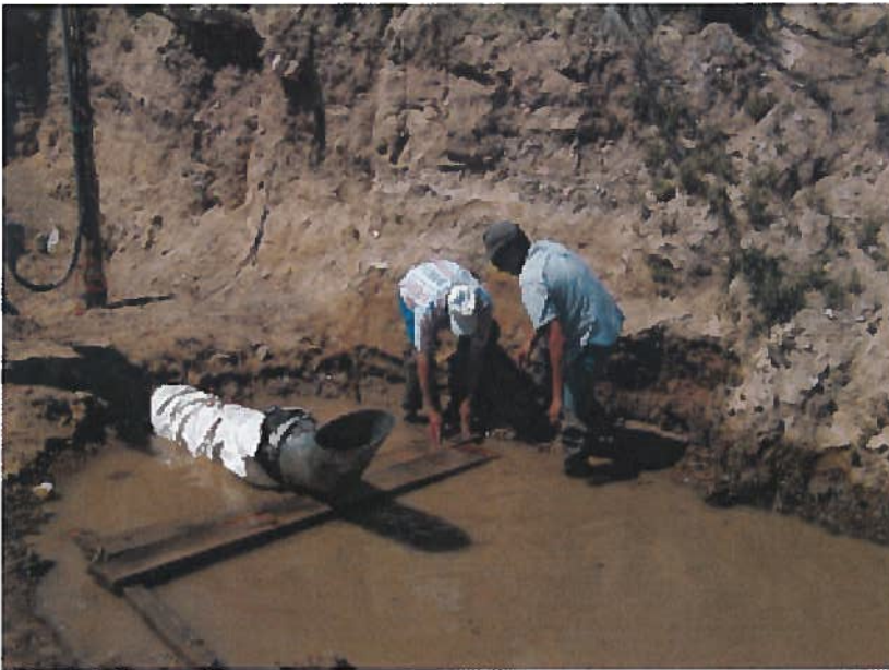
Figure 6. Scott King and Jerry Udy supporting the flow meter.
