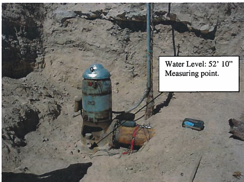
Figure 2. Close-up of Rosco Ward's POD. Originally measured with the Fuji Flow meter. We had a difficult time getting a signal because of the condition of the discharge pipe. Most of the readings were abnormal. The average flow was 2699 gpm, maximum flow 2752 gpm.
