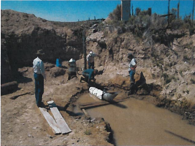
Figure 5. Rosco Ward, Scott King and Jerry Udy (Raft River Rural Electric Co-op, Inc.) installing the Sparling Propeller Meter.
