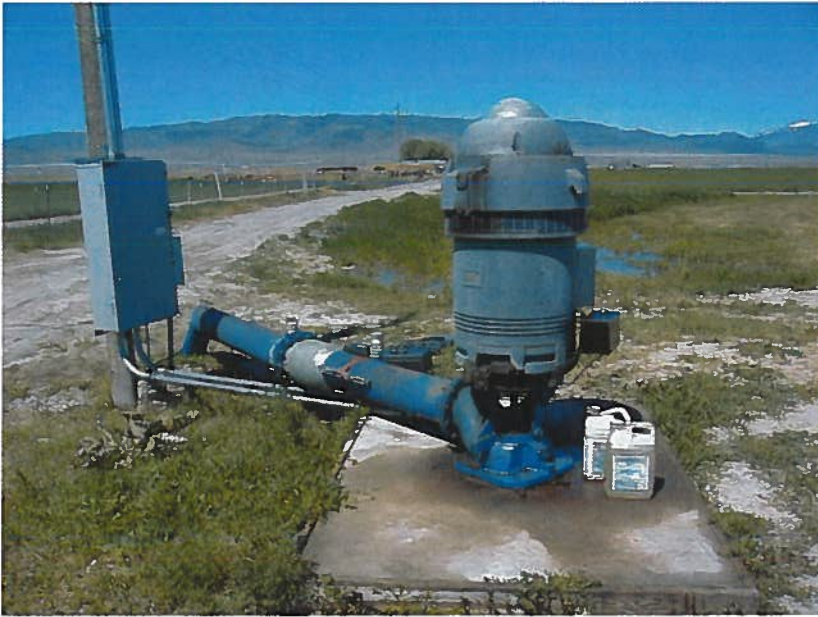
Figure 9. Average flow measurement 1297 gpm or 2.89 cfs. Looking westerly.
