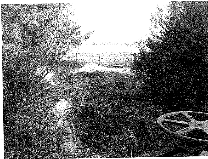
Figure 4. Photo at Location 1 looking east along the ditch at the north side of the property
