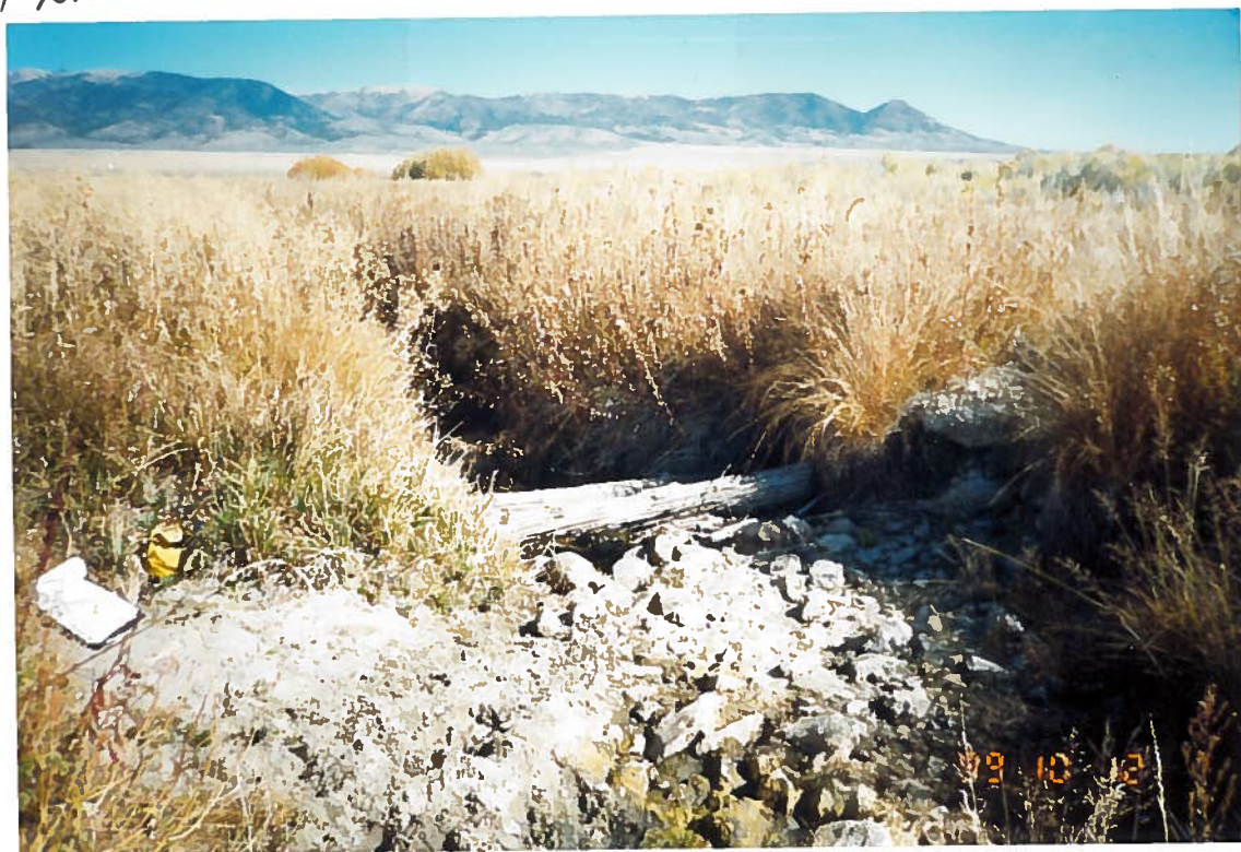
Upper Cove Creek Diversion in Section 25 GPS site R101220A NE NW SE
