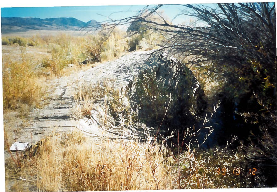
↑ Cove Creek diversion - signs of extreme erosion. Soil Conservation designing new diversion R101219C NE NE SE SEC 25
