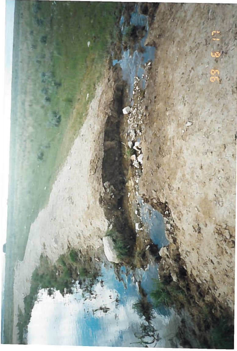
Pond Embankment Breach & Flooding To North
