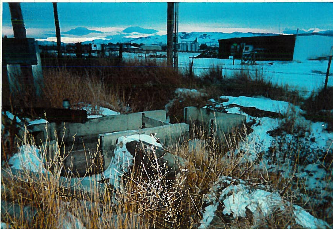
Photo 6. DIVERSION WORKS FROM CASSIA CREEK TO THE CEDRIC TAYLOR PROPERTY. LOCATED IN THE SW CORNER OF THE NWSE SECTION 1.
