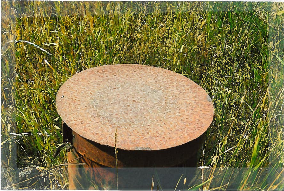
16-Inch Cased Irrigation Well
