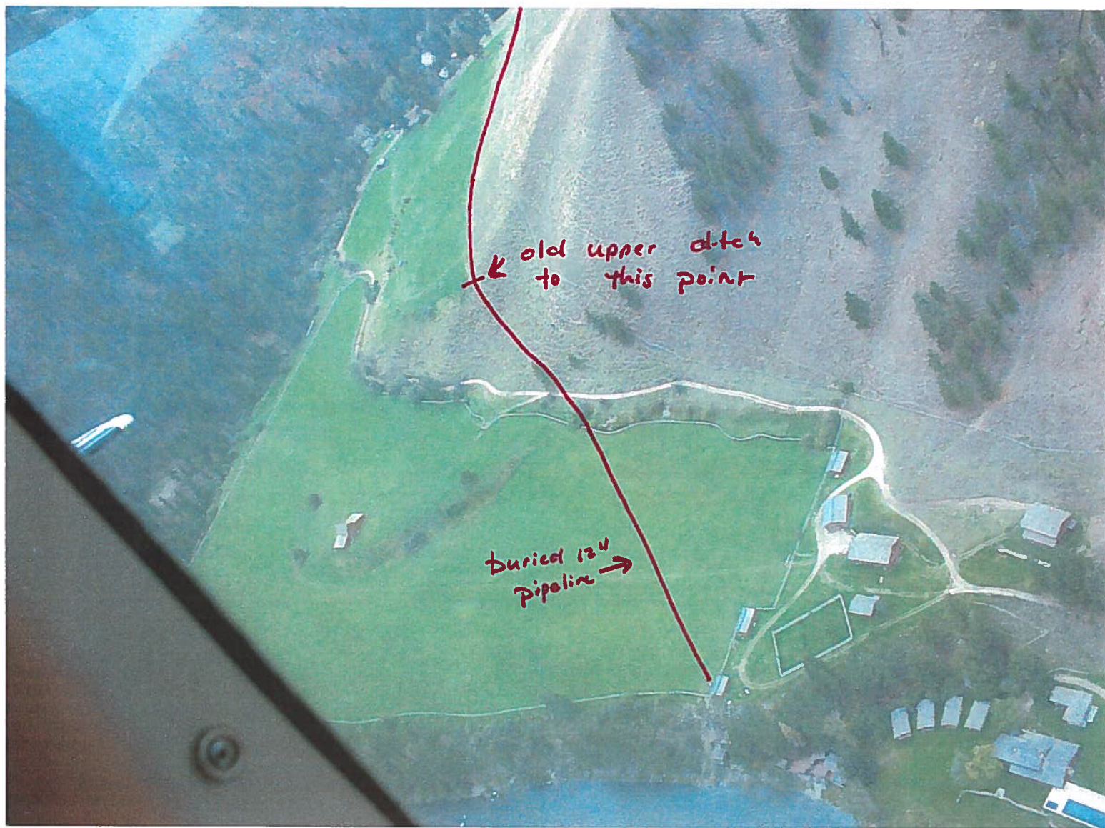
Lower portion of old upper ditch and location of 12" pipeline to hydro plant and sprinklers for hay.
