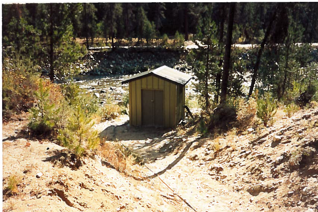
Looking east at pld on Johnson Ck. Pumphouse is seen.
