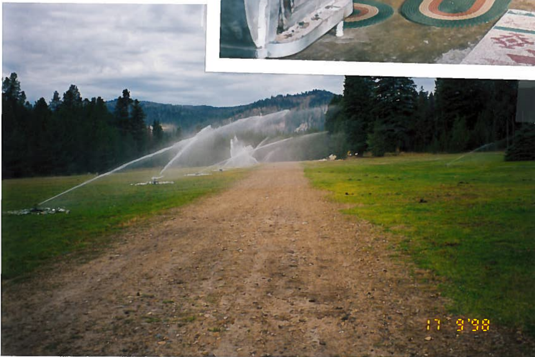
1 acre irrigation with 14 sprinkler (5/16" nozzles) (area directly around the lodge and upper west end of air strip)
