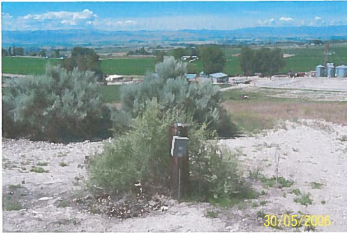
63-9132 Glen Mossel's well at 2295 A.P. Road 325' deep, 34" above ground, 8" casing, 93' static
