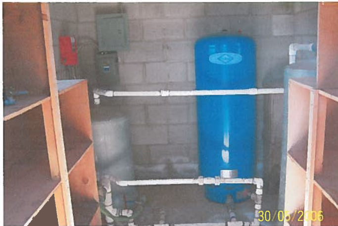
30 psi, challenger tank, red jacket pump 3Hp 1 1/2" discharge No longer belongs to Van Slyke sold in 2005
