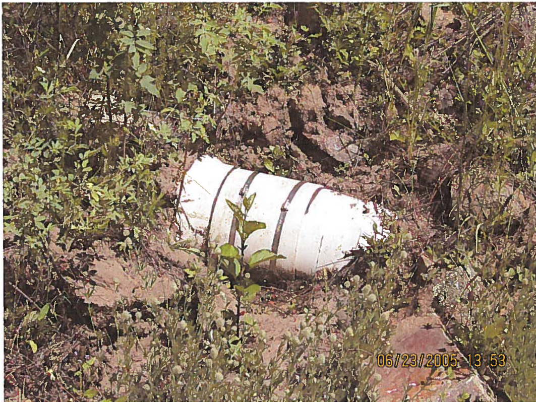
Photo 3: Ten inch PVC conveyance pipe.
