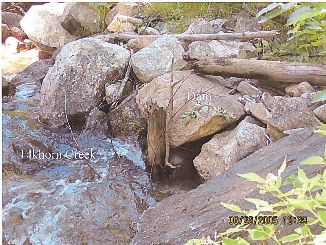
Photo 1: Rock dam at POD.
