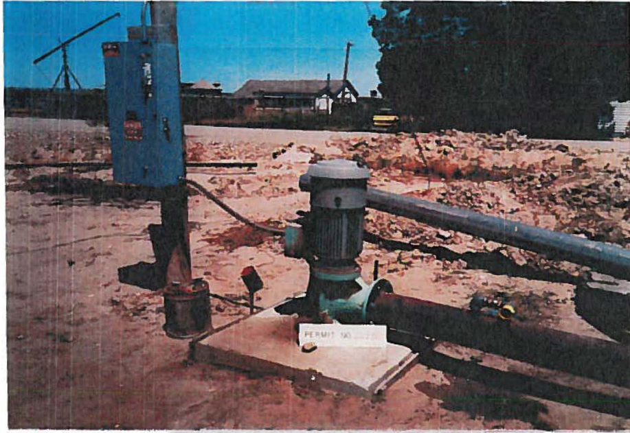
well + 20 HP pump T4N R3W sec 6 NENENE
