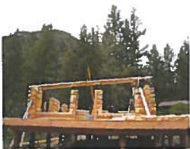
The logs are tied together with the framing of the front windows.
