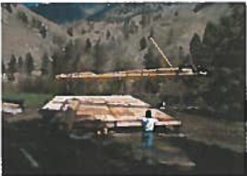
Helicopter sets the first row of logs directly on the foundation platform.
