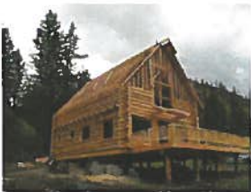
The cabin takes shape as the roof is secured to the log structure.
