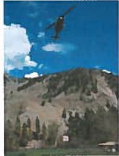
First load of a stack of plywood is delivered to Taylor building site.
