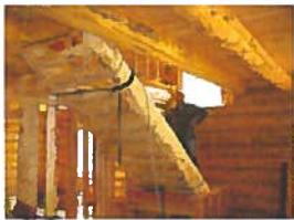
The stairway was constructed of half logs and secured.
