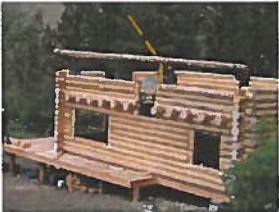
The portable crane which came in by airplane was the only way to set these heavy logs.
