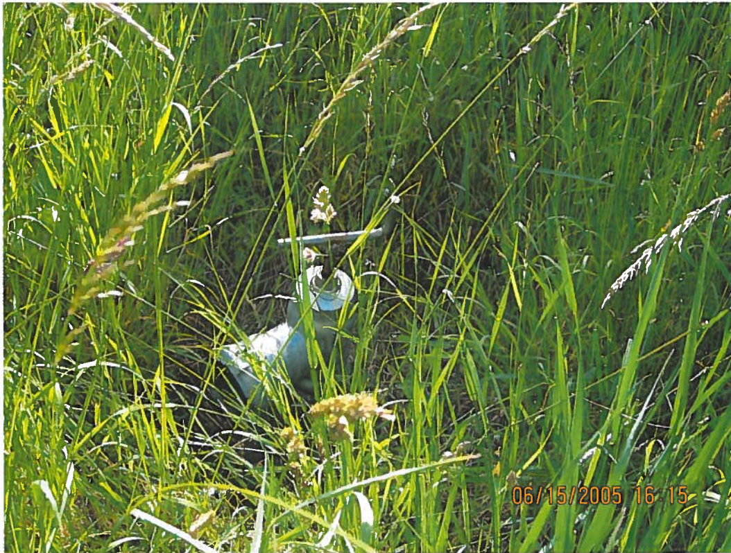
Photo 3: Riser at point 'A' on Photo-Quad Map.
