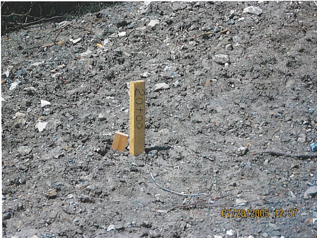
Photo 3: Grade stake for new ditch.
