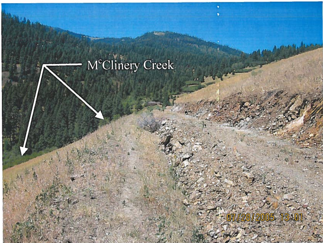
Photo 2: Looking northwest over partially built pad for new ditch.
