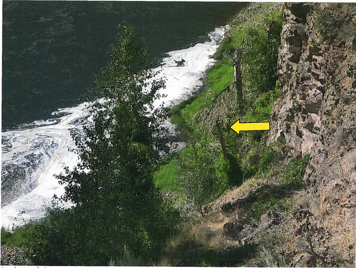
A view of the pump area from above. The foamy portion of the water is the general location of the pump when it was in use. The pump currently sits under the trees at the left of the picture. The power pole is indicated by the yellow arrow.
