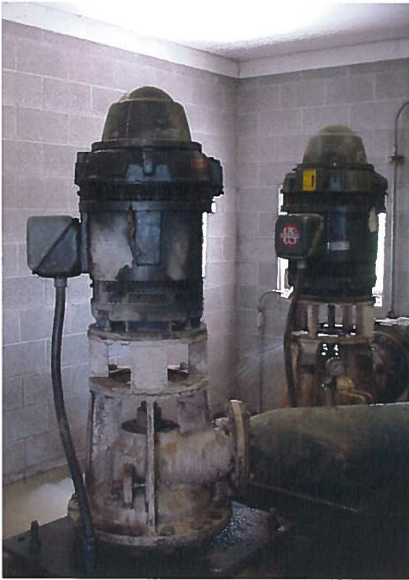
Pumps #3 & 4 - 10" pipeline to center pivots
