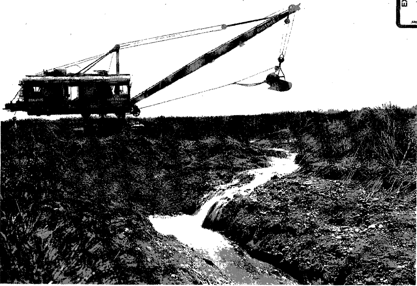
P4-100-3348 Electric dredge excavating Purdam Slough Drain on Lemp's ranch. Arrowrock Division, Boise Project, ID. USBR photo by Walt Lubken. Jun 22, 1914.
