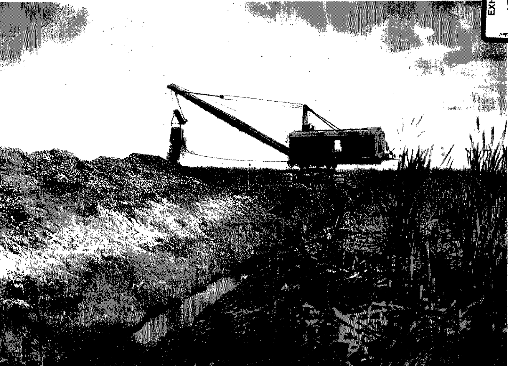
P4-100-3347 Electric dredge excavating Purdam Slough Drain on Lemp's ranch. Arrowrock Division, Boise Project, ID. USBK photo by Walt Lubken. Jun 22, 1914.
