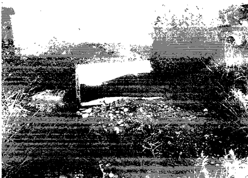
Photograph 2: Trapezoidal flume appears to be Plasti-Fab model 12" x 45" SRCRC.
