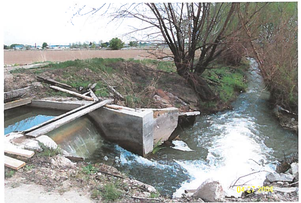
Spill off of lateral
