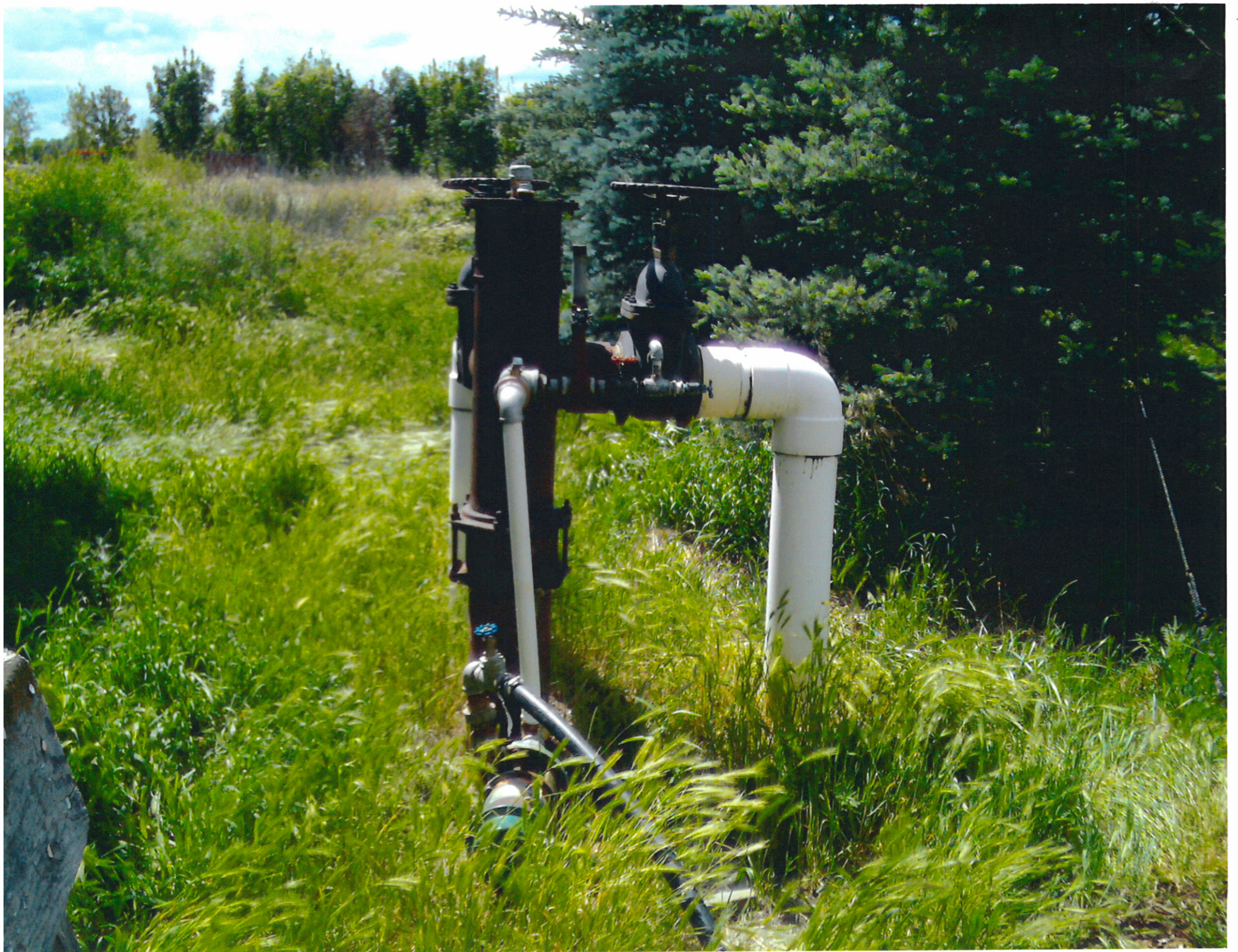
Figure 1: A photograph of a water control structure, possibly a weir or gate, situated in a grassy field. The structure features a vertical black frame with two large, white, curved gates. The gates are partially open, allowing water to flow through. The background shows a dense line of trees under a blue sky with clouds.
