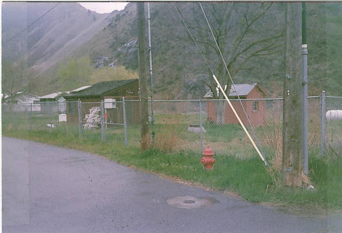
Pumphouses Looking NE C4
