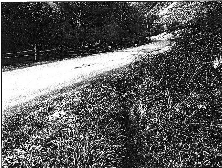
Figure 2. Downstream side of the canal culvert under the Squaw Creek Road. The canal joins with the main canal that flows through the overpass just outside the photo.
