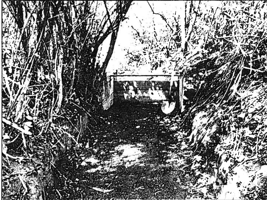
Figure 4. Downstream side of the Squaw Creek headgate.
