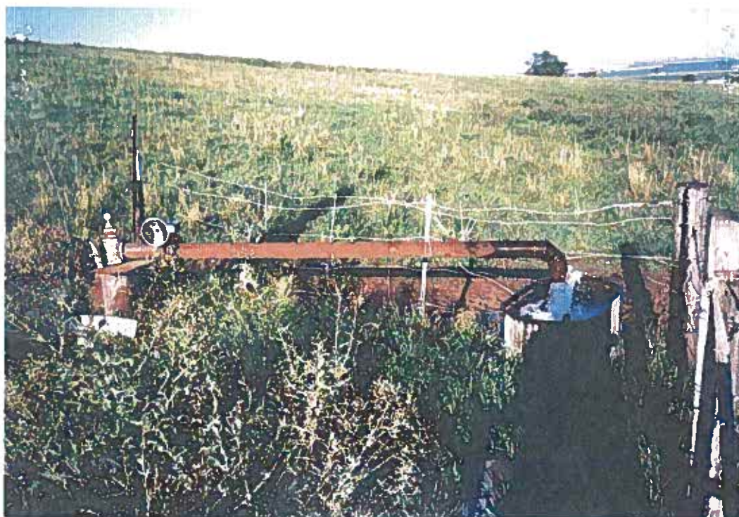
P.D. Looking West
