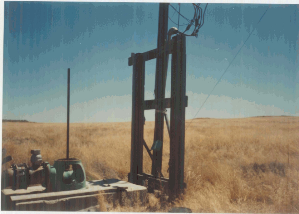
#1 P/D - well site, motor removed
