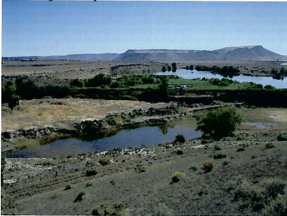
Photo taken of central section of impoundment as seen from White Butte.
