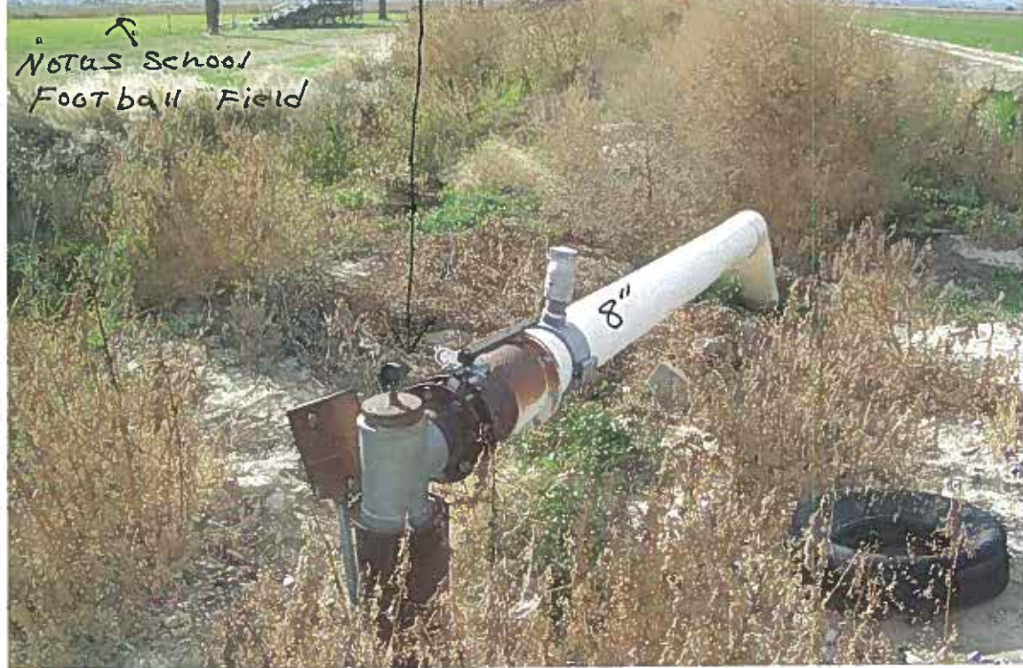
Pic #1 Point of Diversion
