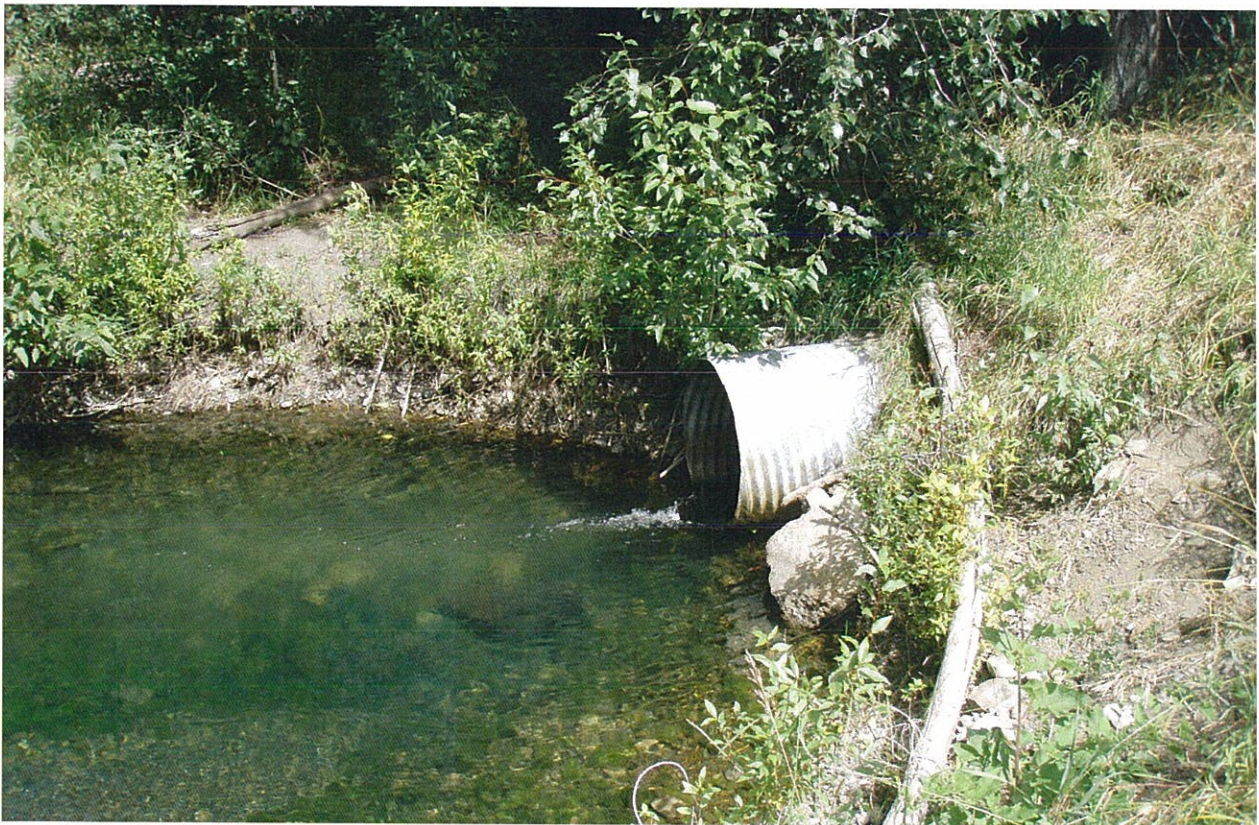
BELOW: View of the downstream end of the low level outlet below Dollar Road.
