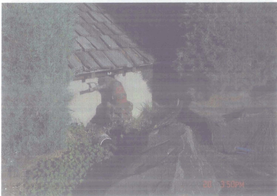
Pump House At Pond III that Irr. Stony Park GPS 43°34.620 - 11610922
