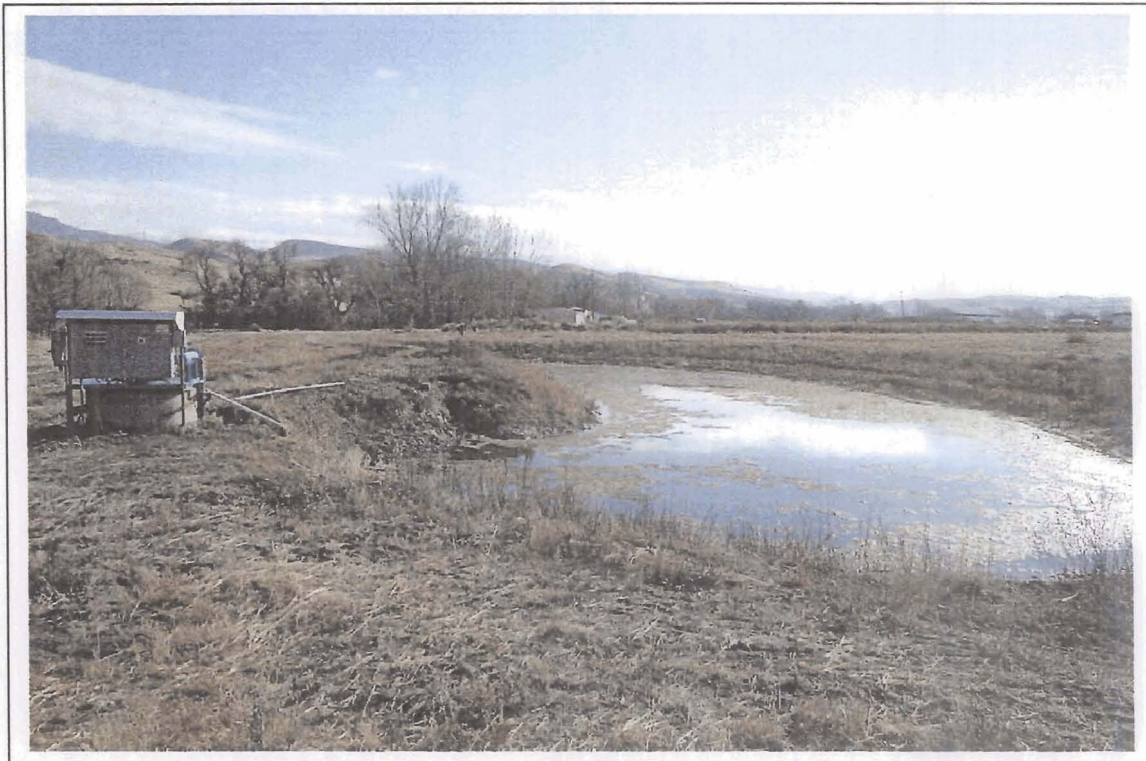
Photo 7: Distribution pond & pressurized system, view is to the east. See attached measurements. The pond has 5.17 AFA volume MAX. The well water is supplemental to surface Dry Creek right and thus the MAX combined flow is 2.78 CFS. (2.78)(1.9835) = 5.51 AFA.
