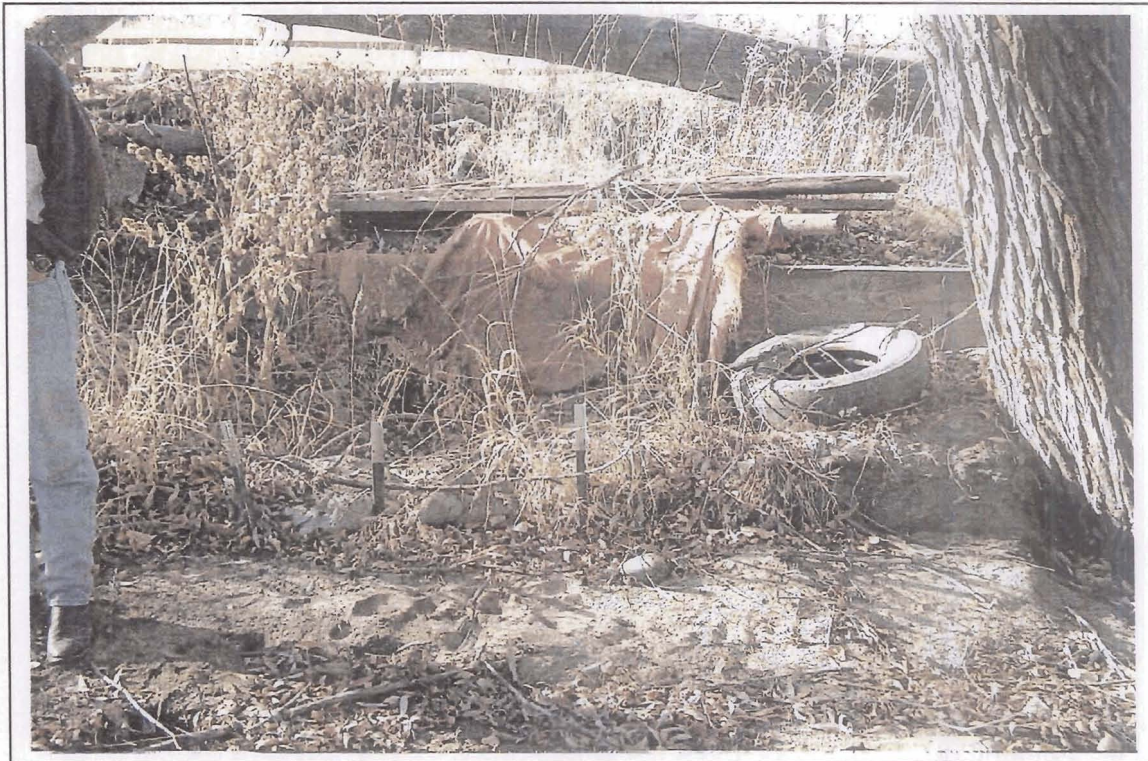
Photo 1: 63-4849, Field Exam 11-14-02: Located in the SESENE, S31, T05N, R02E. GPS location. This is one of the old system's points of diversion that is still being used. This is the South ditch from Dry Creek. Discharge west into a south gravity flow ditch. Pumps were used from other ditches to deliver water to area's not reached by gravity irrigation. A north ditch is no longer used for this right.
