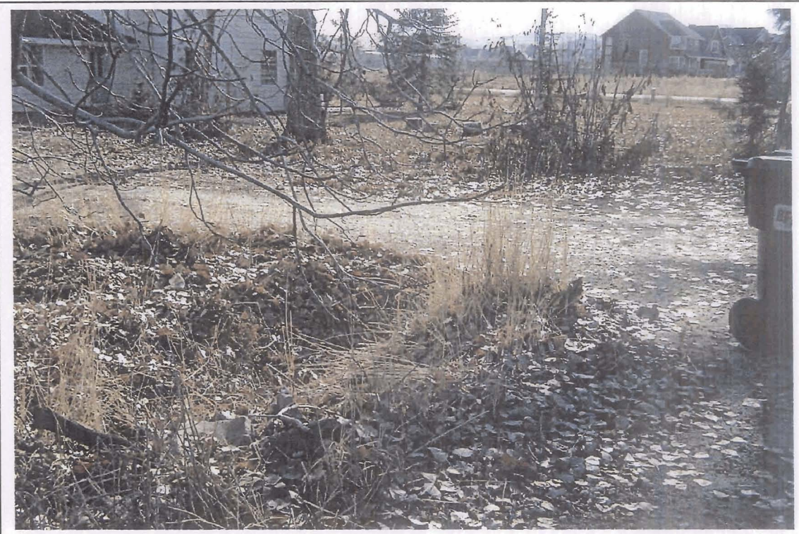
Photo 3: Culvert with gravity flow from Dry Creek on East side and under McFarland Creek road.
