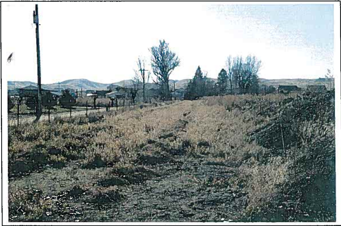
Photo 5: View to South along McFarland Creek road where underground pipe carry Dry Creek water to distribution pond.
