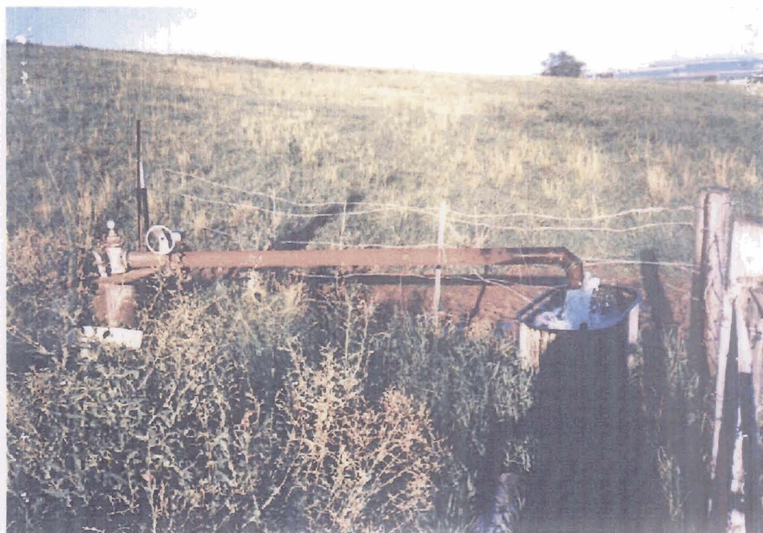
P.D. Looking West
