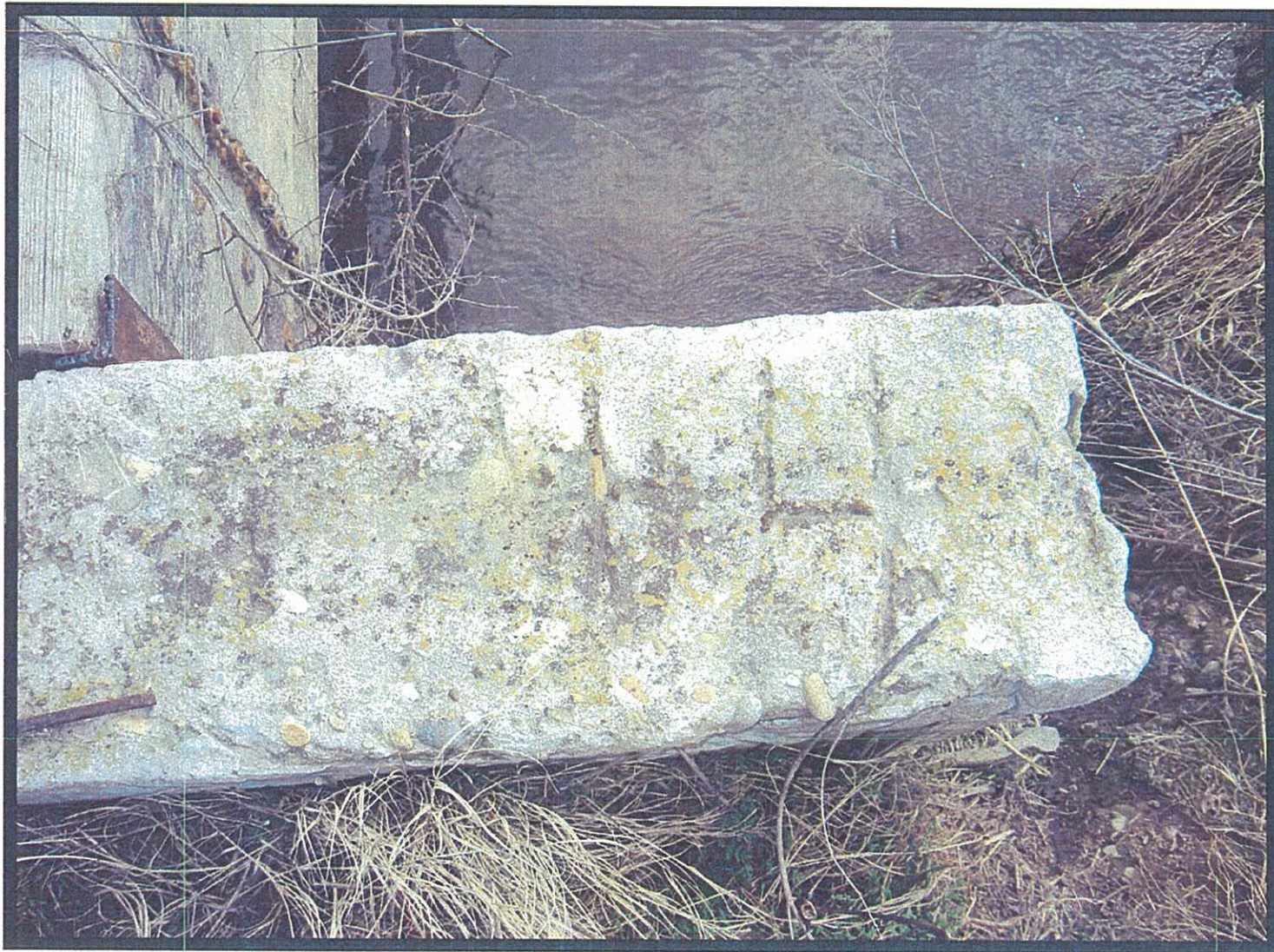
1944 Date of Reconstruction for Diversion Structure to Upper Haas Ditch
