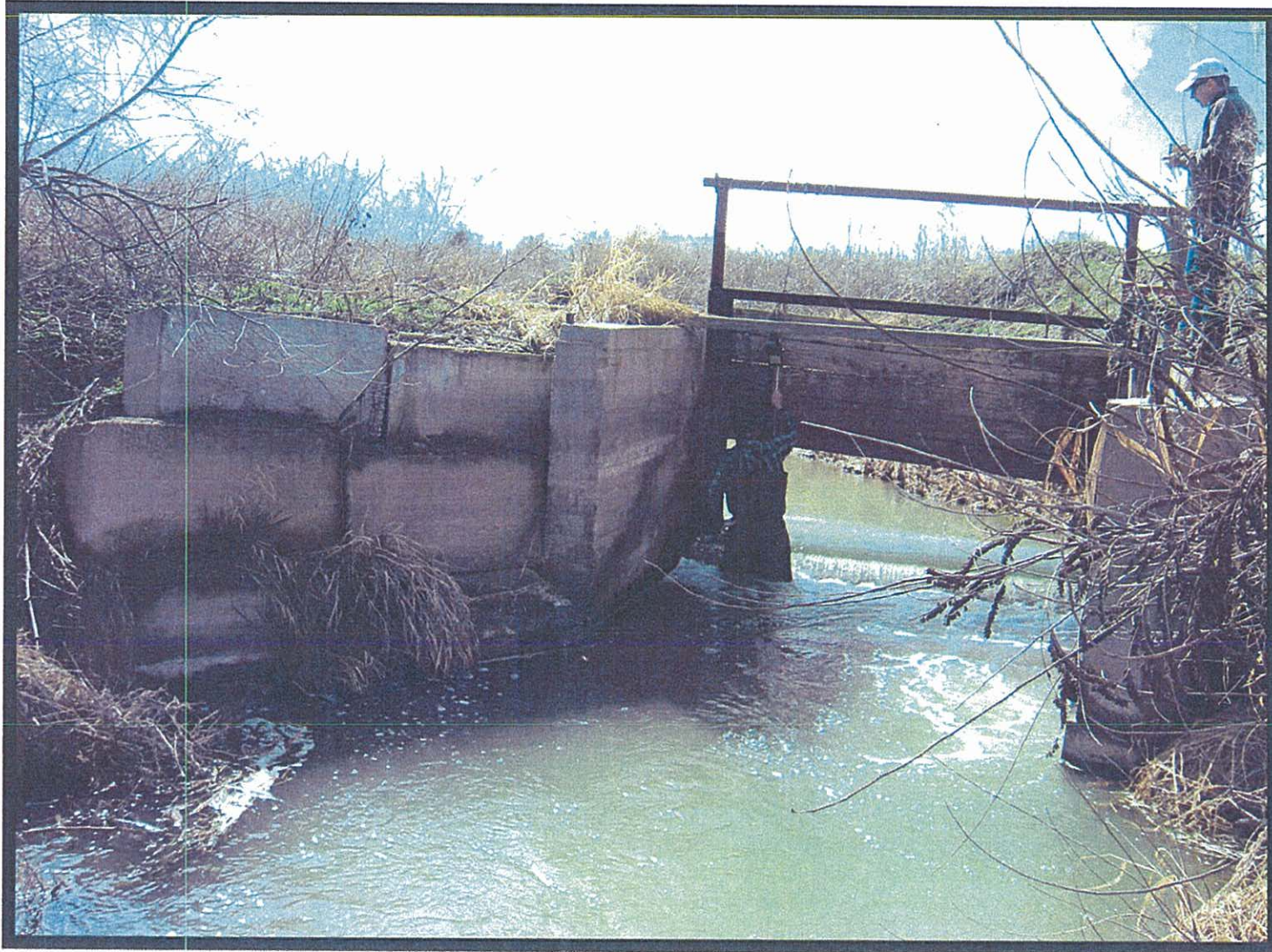
Diversion Structure for Upper Haas Ditch (photo taken 3/3/2010)
